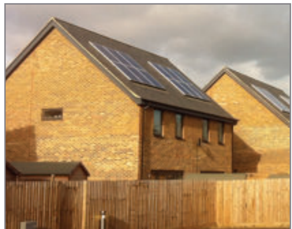
PV array on rear elevation of dwelling in Whittlesford, included in the occupant interviews.
